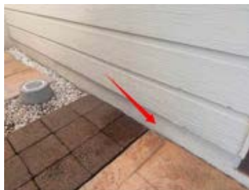
Possible Entry Points for Termites into Monolithic Slab
